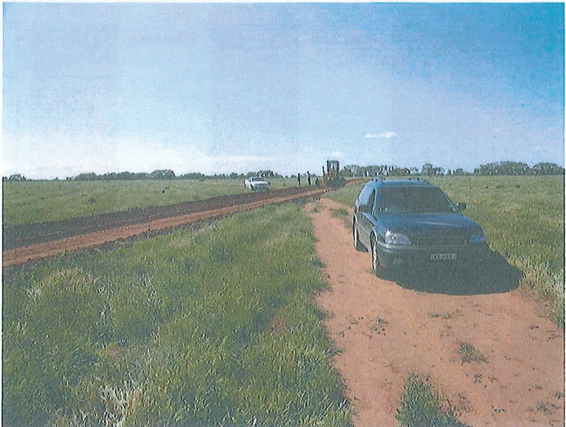
Figure 30. Road grader mechanically scraping transect T2.
